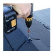
Position the Fast Union Clip into the slot in the top of the Fast Union and secure with the Fast Drive Screw.
